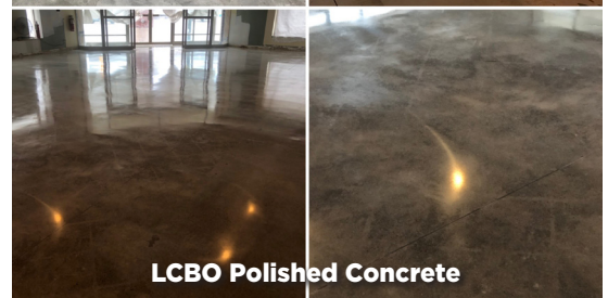
Polished Concrete with Aggregate
