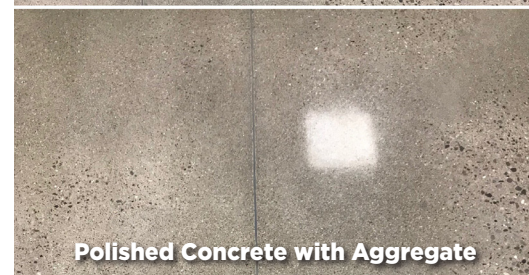
Polished Concrete Exposure 3 with Waves
