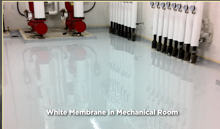
Waterproof Membrane in Mechanical Room
